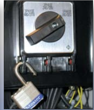
The three-position voltage selector switch is lockable.
